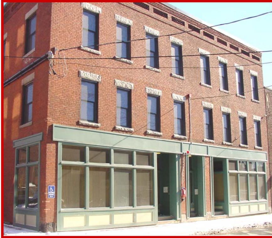
“The Irving House” Framingham, MA
